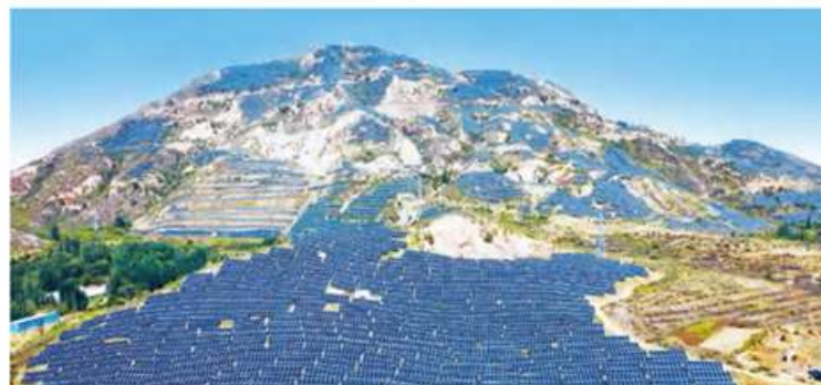
Location: Croatia Capacity:120kW/200kWh
