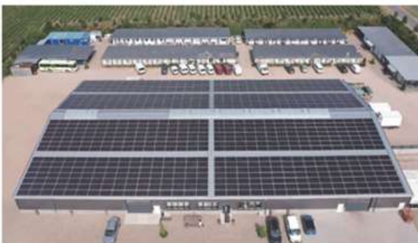
Location: South Africa Capacity:1MW/1.3MWh
